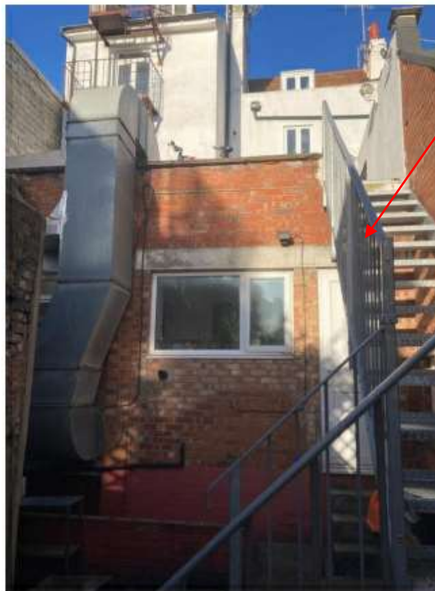
Stairs to existing dwelling
